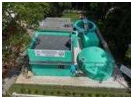
360 KLD STP at General Hospital, Thrissur
